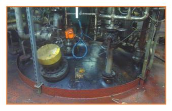
Based on extensive experience in such applications, Hycontrol engineers were confident their ATEX compliant VG7 radar level measuring system with drop antenna and DiFoam non-aqueous foam probe and control system would meet the dual challenge of accurate tank contents measurement and improved foam control with reduced de-foamer consumption. As
